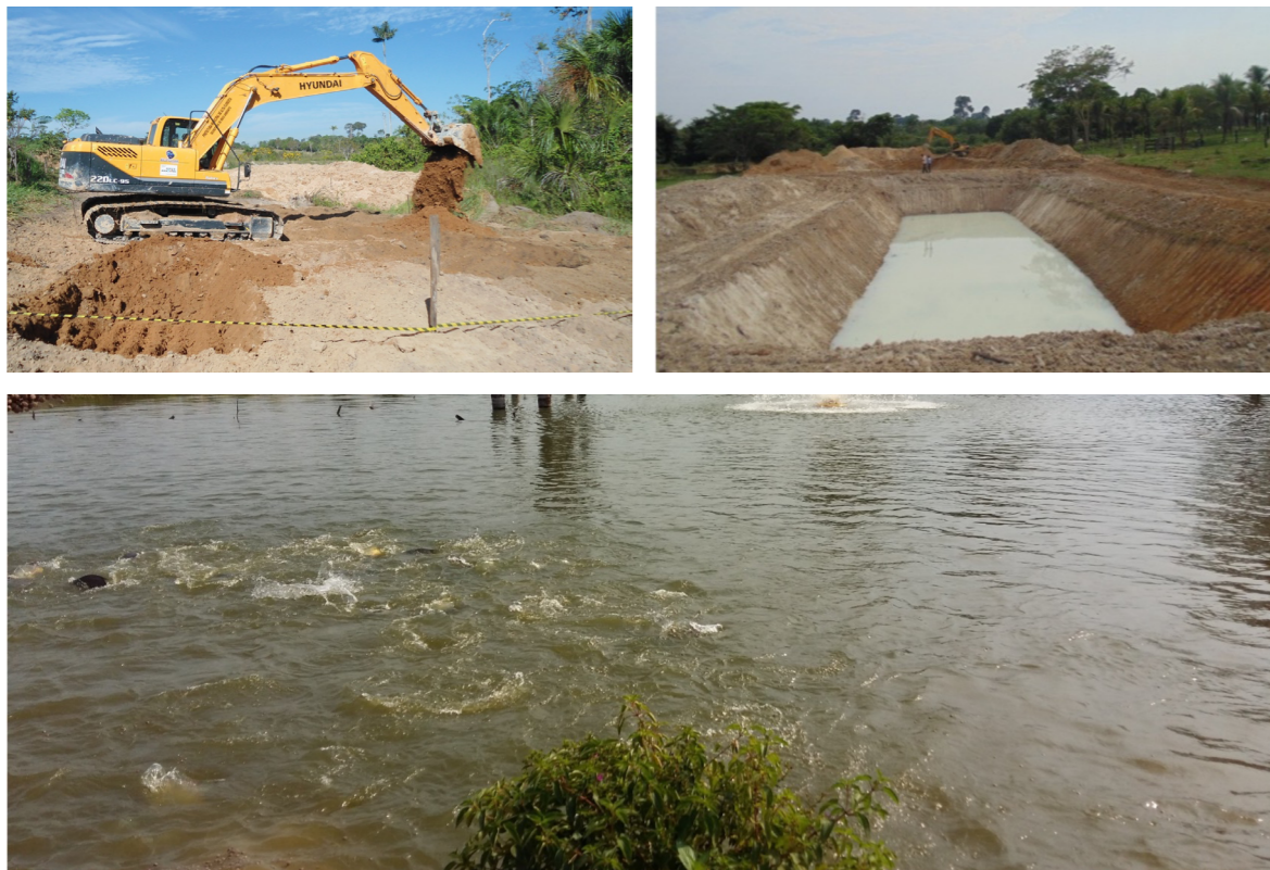
Figure VII: Construction of fish farming tanks in Alta Floresta
