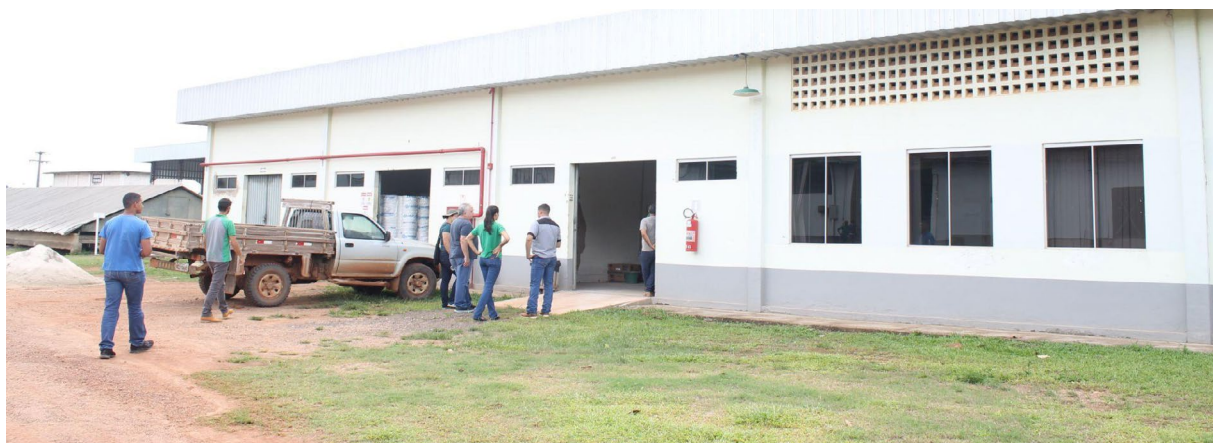
Figure V: Oil processing plant rebuilt with additions to original project after fire in 2015
